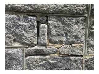
We ended up with fresh mortar filling in the entire depth of each granite block:
