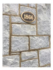
The finished area surrounding the front entry is easy to distinguish. Over time the slightly darker brown new mortar will lighten to match the old mortar.
