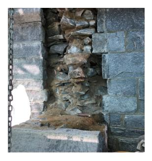
Each ashlar stone was numbered and arranged in tandem along the scaffolding deck while the underside was washed and prepared for the rebuild. As one of the masons rather modestly remarked, "It's somewhat like reassembling a jigsaw puzzle." For more pictures and description of this ongoing journey, please visit our dedicated website and blog: <a href="https://www.set-in-stone.org/">www.set-in-stone.org/</a>
