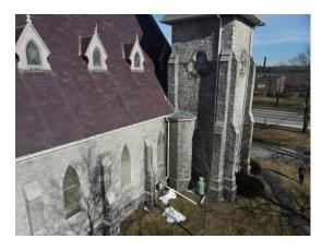
Tucked around the back, away from Central Street, and facing Pleasant Street, the West tower wall is not readily noticed. But a close look at it (see next picture) reveals major areas of missing mortar, cracks, and shifting of stones. The clover-shaped trefoil window also has open areas around it. We've had the window patched from the inside – a temporary and partial fix. All of this leads to water ingress: the biggest enemy of any building.
